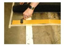
5- remove protective liner and recover with SW3270(E):
